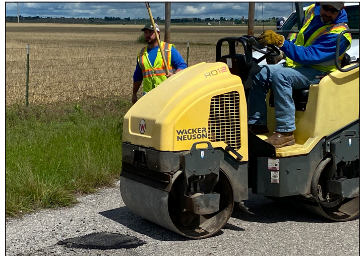
Pictured: Jesse Trejo, Braydon Horn and Brett Holding work on Shepard Road north of Britton, patching potholes and rolling out fresh asphalt.
